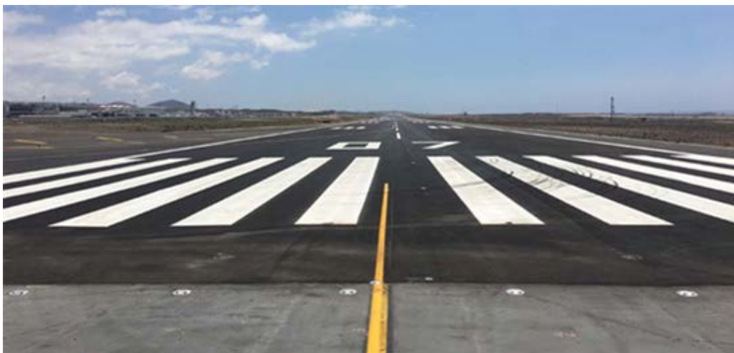
Resurfacing of Tenerife South Airport Runway
