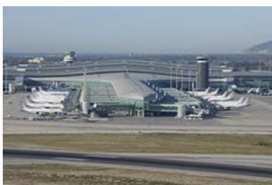
Picture 2. Apron – Barcelona-El Prat Airport
