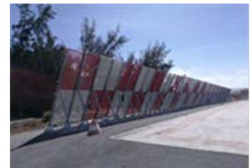
Picture 20. Blast fence. Gran Canaria Airport
