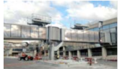
Picture 28. New airbridges at Malaga Airport
